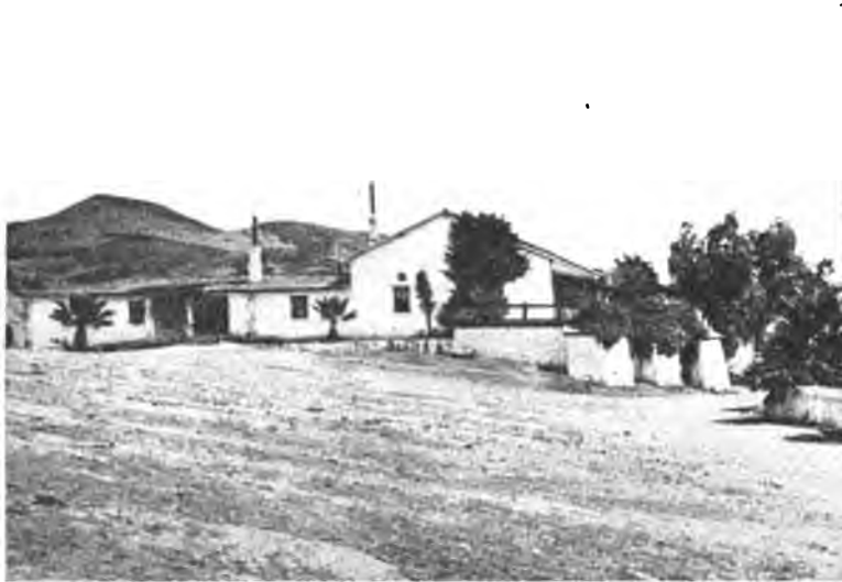
O'NEILL RANCH HOUSE (LOOKING SOUTH) BUILT BY PIO PICO IN 1820.
